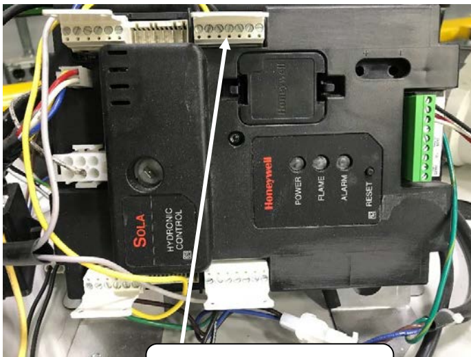
Disconnect sensor harness from control board
