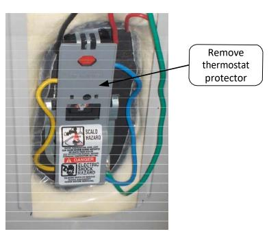
6. Disconnect wire leads from element(s) terminal block.
