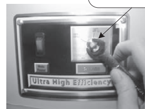
Remove retaining nut
